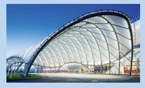
various ways to alter its transmittance to control the internal environment (Fabritecture, 2017). ETFE has a low energy manufacturing and transportation process (due to its lightweight). It performs well in earthquakes due to its elasticity and does not allow flames to spread in the event of a fire due to its ventilation and self-extinguishing qualities (Lynch, 2019).
